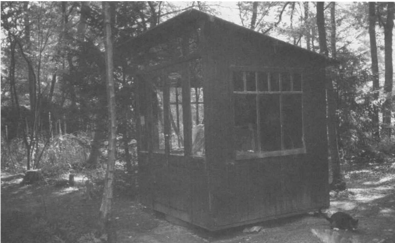
A small structure on a rotating base that could follow the sun. These little houses were often used by tuberculosis patients, hence the name "TBC hut."
